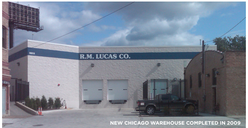
LUCAS CORPORATE HEADQUARTERS, RESEARCH AND MANUFACTURING FACILITY IN ALSIP, IL OPENED IN 2015
